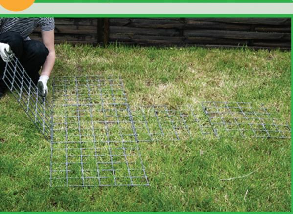
Unpack the gabion, ensuring all sides are properly unfolded and ready for assembly.
