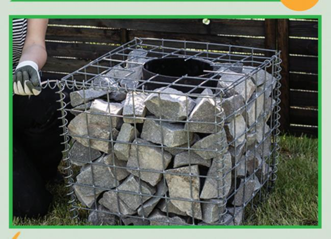
Close the lid and join the corners with a helical, repeat this process for all corners.
