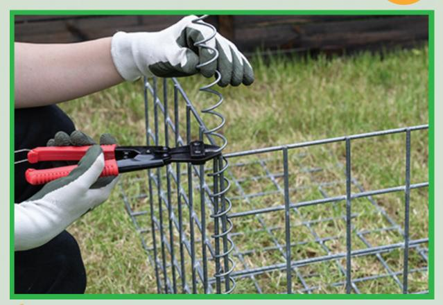
Measure the dimensions of the gabion panels and cut the helicals to match accordingly.
